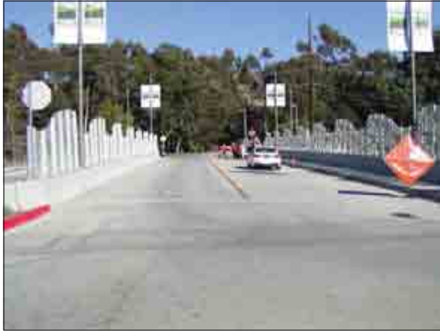
Looking east at the bridge over La Cienega Boulevard
