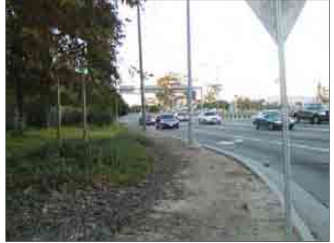
Looking northeast at the northwestern corner of La Brea Avenue and Stocker Street
