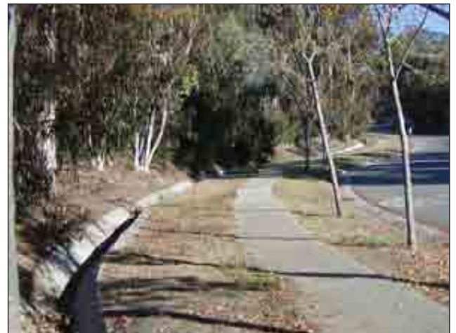
Sidewalk along access road
