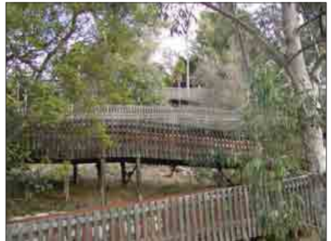
Looking east at the existing trail within Culver City Park
